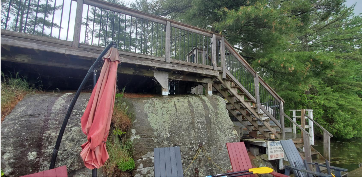
Site Photo 3: View of Decking and Exposed Bedrock
