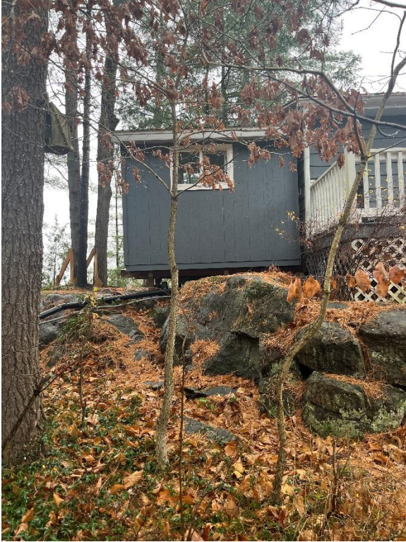
Site Photo 4: Pumphouse Elevation Facing Burma Lane
