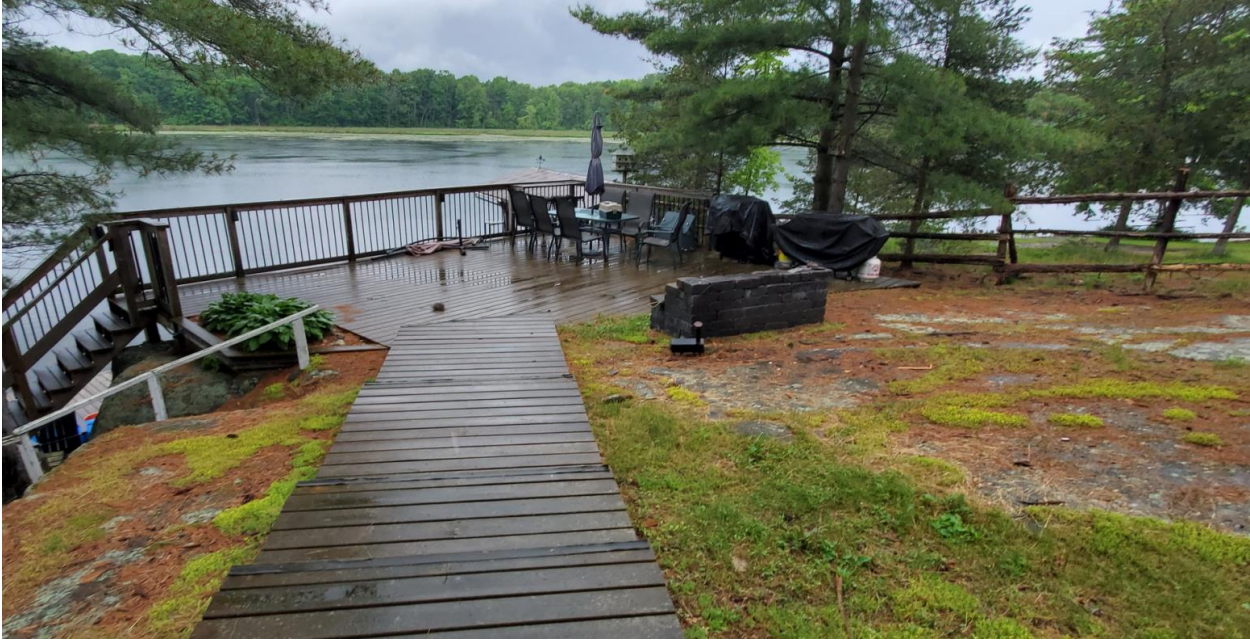
Site Photo 2: View of Existing Detached Decking
