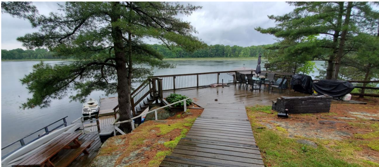
Site Photo 1: View of Existing Detached Decking
