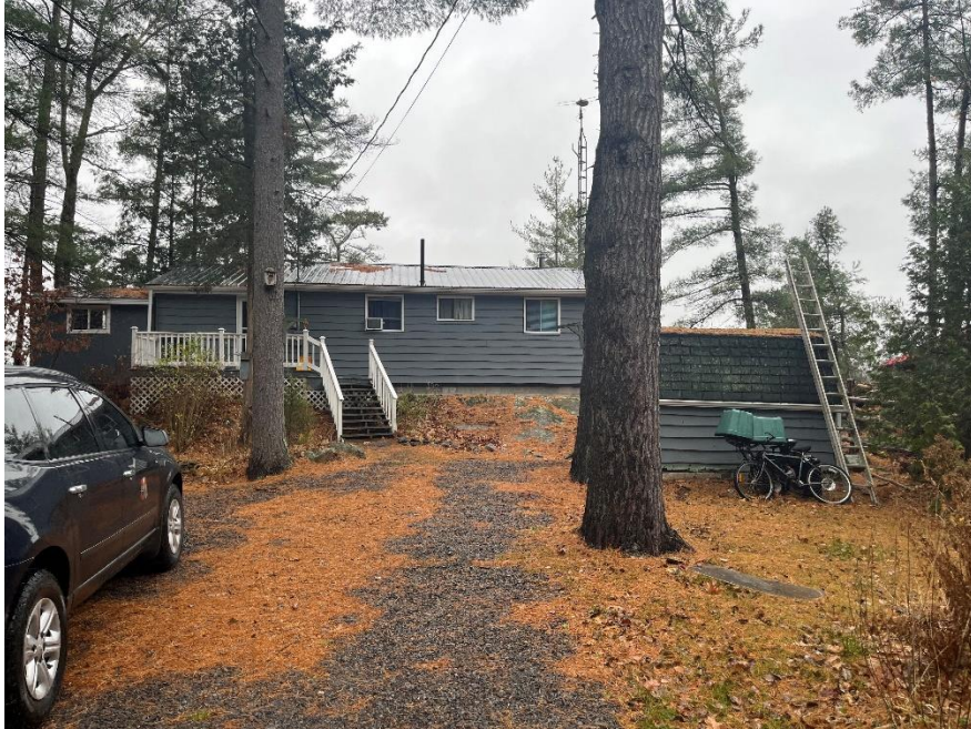
Site Photo 6: View of Existing Dwelling, Shed and Pumphouse from Burma Lane
