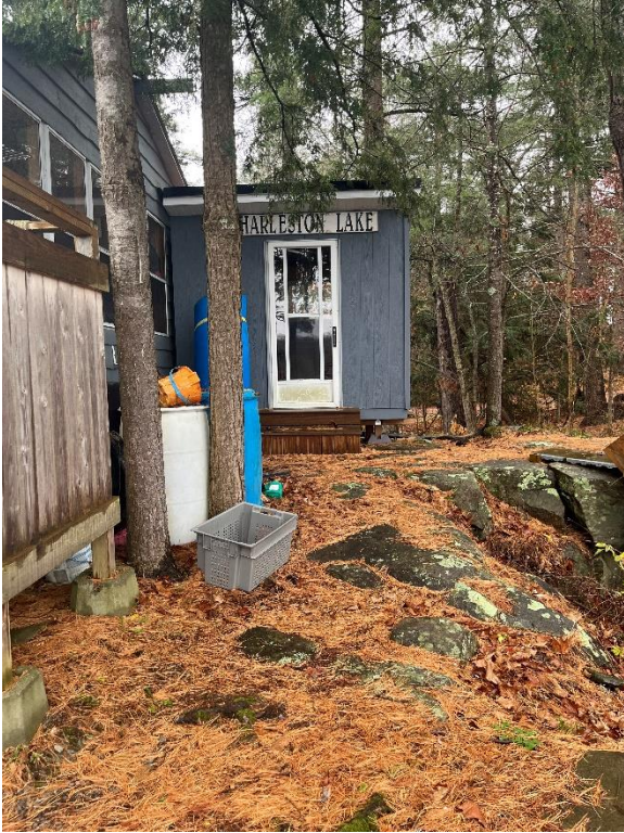
Site Photo 5: Pumphouse Elevation Facing Charleston Lake
