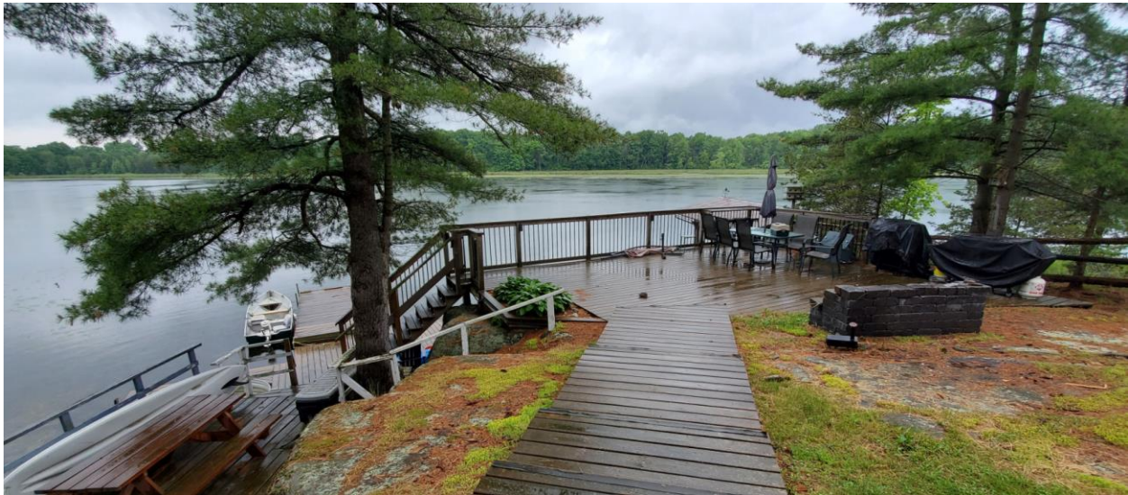
Site Photo 1: View of Existing Detached Decking
